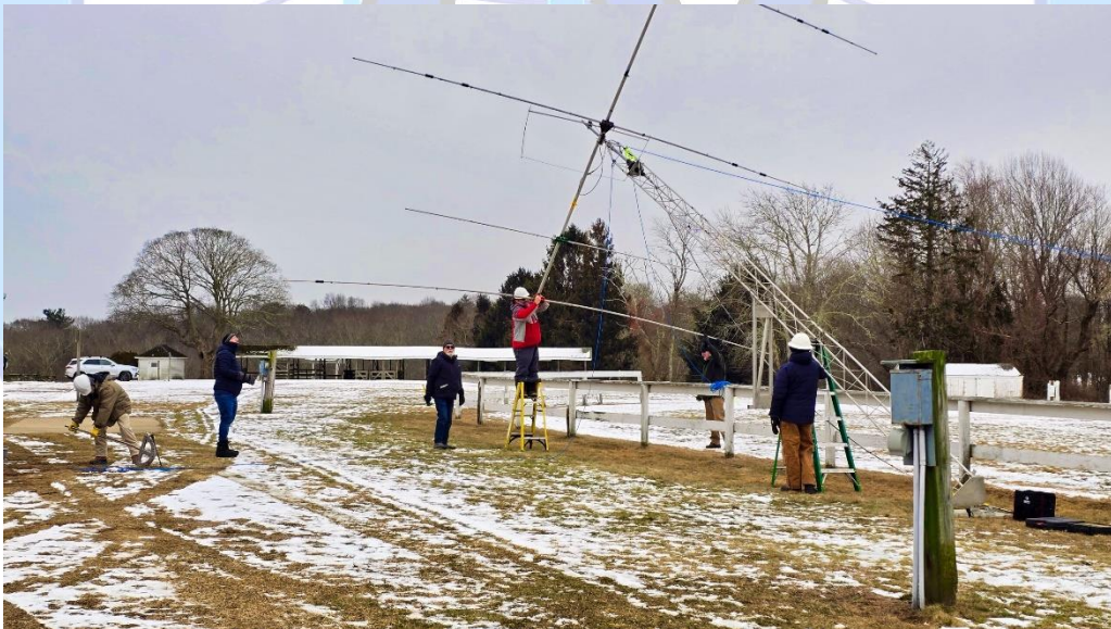
With snow falling tri bander and tower breakdown begins.
