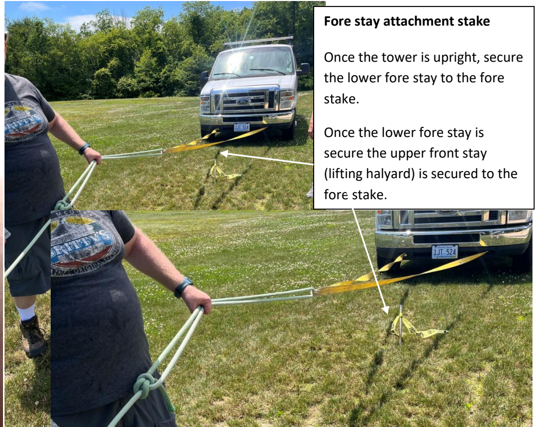
Figure 22 Big White Van (BWV) in position to lift tower. Yellow lifting strap securely hooked to undercarriage and front lifting halyard securely tied to lifting strap. Only the lower front stake is installed.
