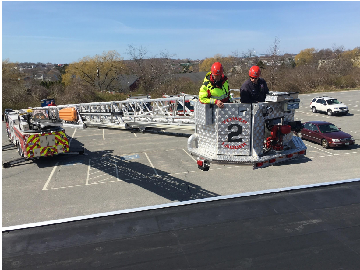
Middletown Fire Department assists in lifting heavy gear onto the roof
