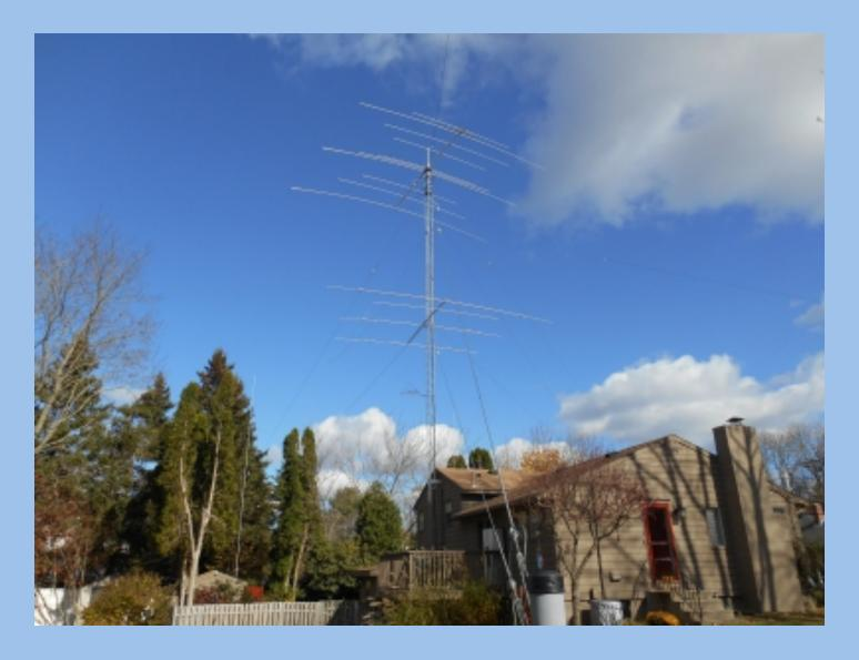
Current antenna farm: Skyhawk at 70'; Cushcraft A4S at 42'; phased with WX0B StackMatch; Inverted Vs on 40 and 75/80 meters.
