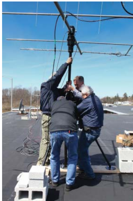
Setting up the tracking antenna
