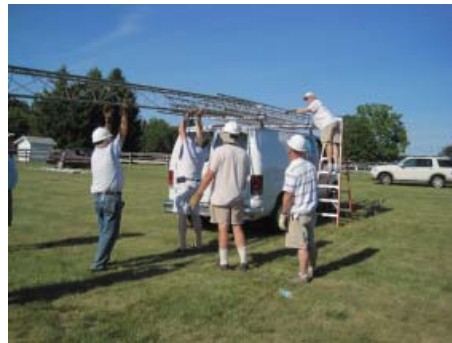
Loading the towers.
