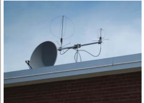
Growing antenna farm.
